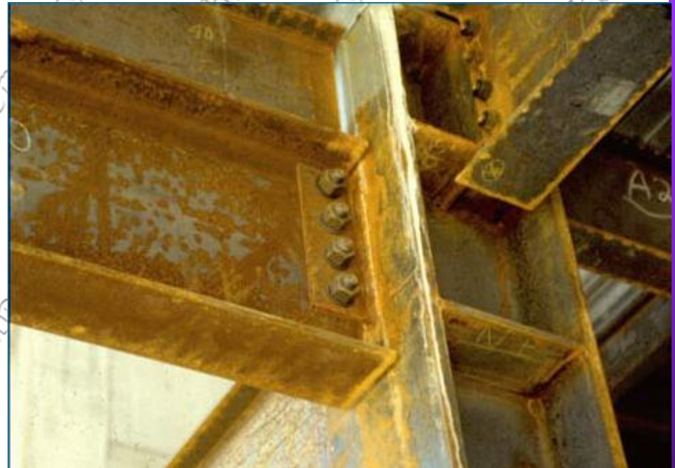
Fin plate beam to column connections
