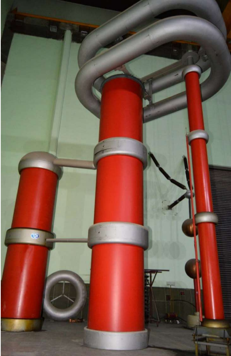
High-Voltage Alternating Current (AC) Generator with a 1 MV Output
